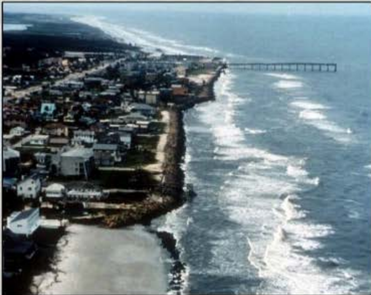
Pre-Initial Construction (circa 2000)
